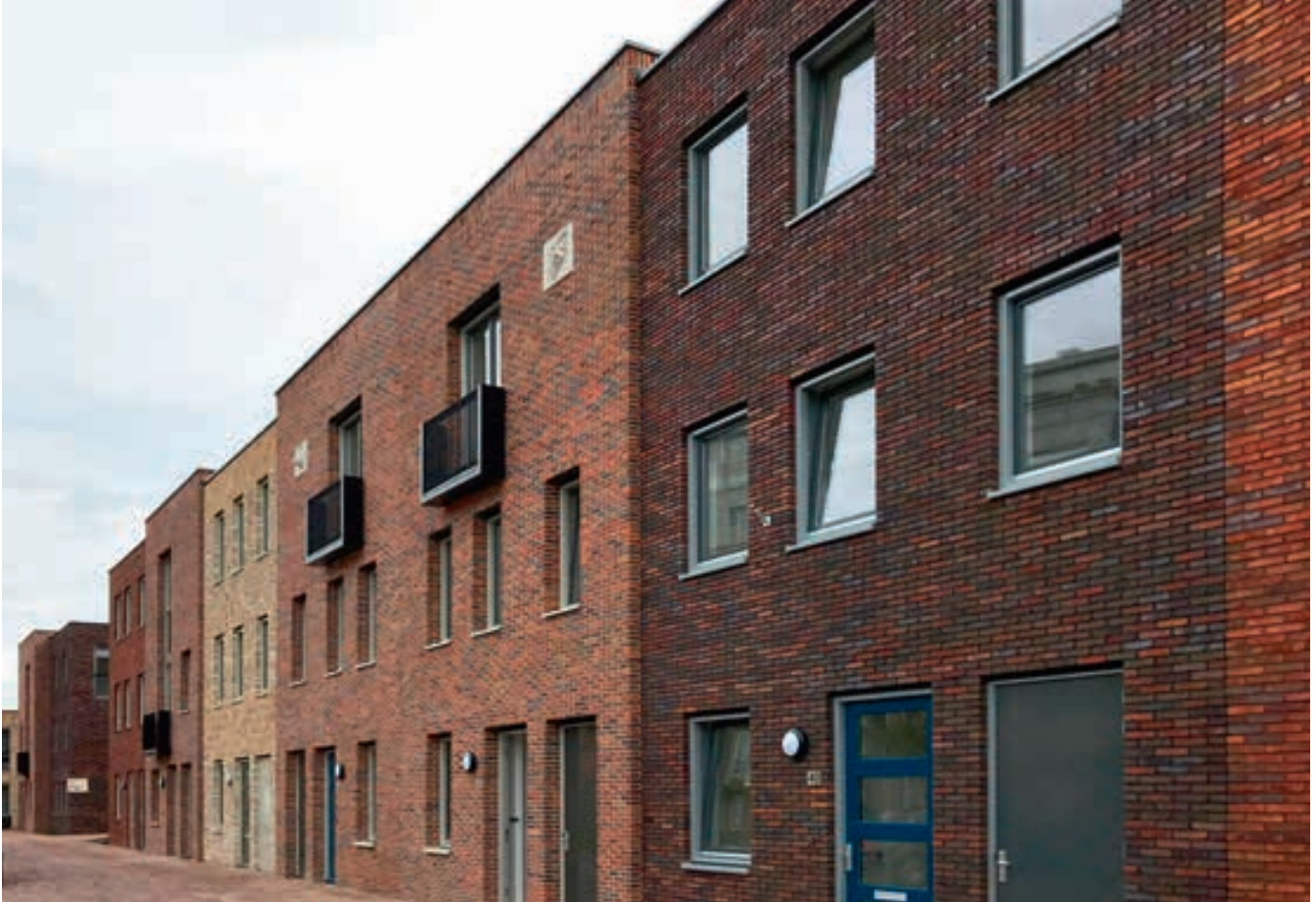
Mix Cumberland Falls WS, Iris Falls WS, Mingo Falls WS, Niagara Falls WS, Patos Falls WS Attika Architekten, Amsterdam
